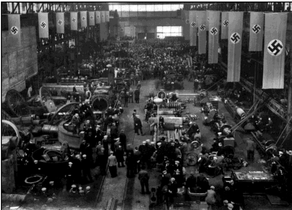
Hagondange plant bedecked by the nazis.
